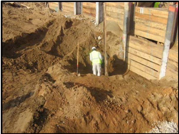
Figure 6: Support of Excavation
